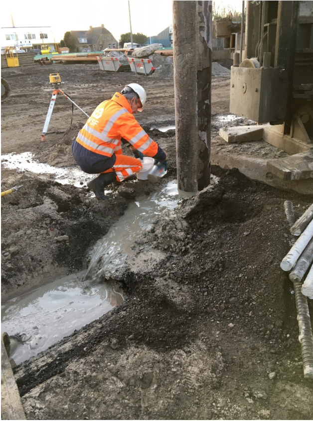
Fig. 6. Sampling of back flow grout
