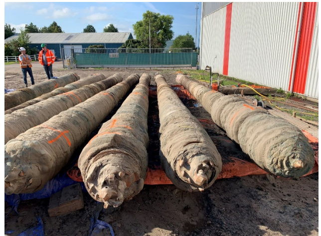
Fig. 9. Extracted piles with screw tip in front
