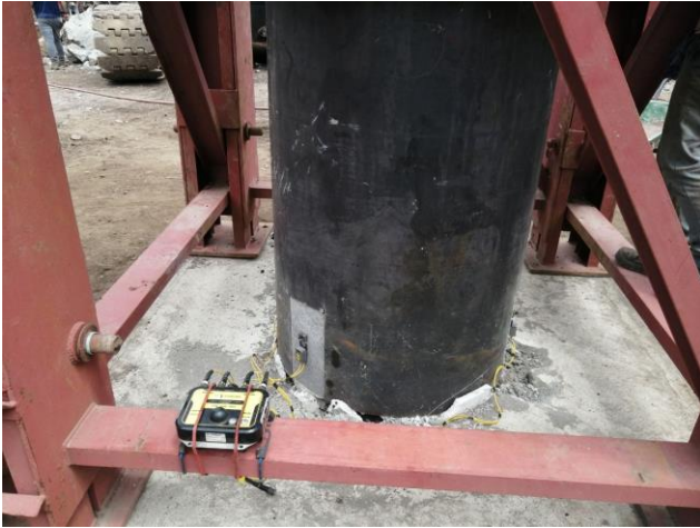
Fig. 3. Set-up for DLT. PDR equipment and sensors on pile, with steel sleeve on head. Ref. Photos from Sectr Tower project.
