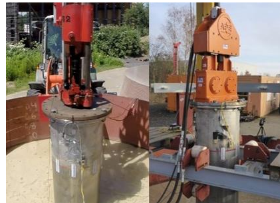
Fig. 2. Impact hammer Delmag D2 and vibratory hammer APE J&M Model 23.
