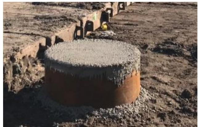
Fig. 5. Extended pile head.
