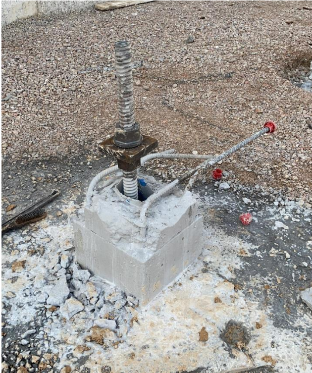
Fig. 1. Precast pile with TITAN self-drilling grouting micropile.
