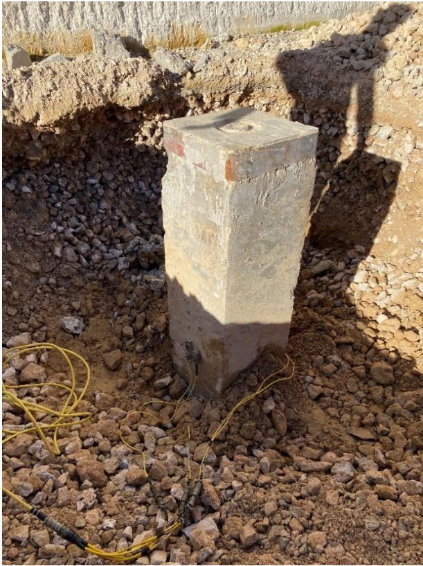
Fig. 3. Pile ready for dynamic load test.
