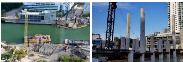
Fig. 6. SR968 bascule bridge over Miami river project site.
