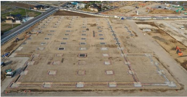
Fig. 3. Example of a construction site of TNF system (at the stage of completion of footings).
