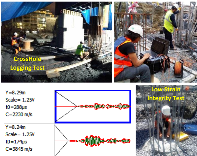
Fig. 8. General views from low strain integrity and crosshole logging test.
