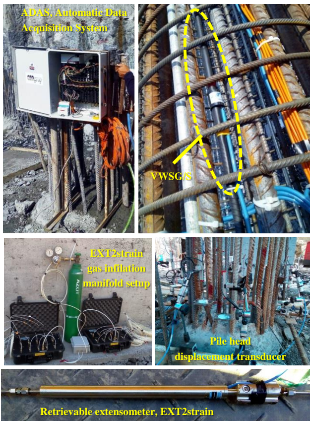
Fig. 3. General views from the instrumentation detail.
