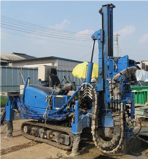
Fig. 1. Construction machine of H-section steel pile.
