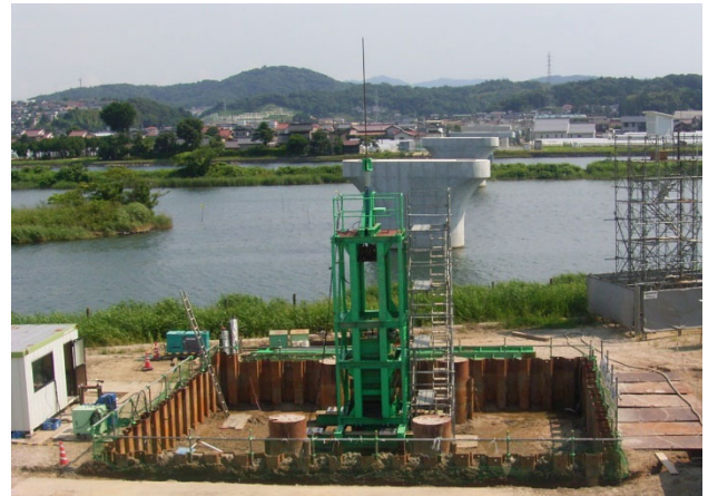
Fig. 10. Load tests conducted at the construction site.
