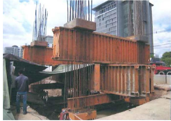
Fig. 8. Static pile load test.
