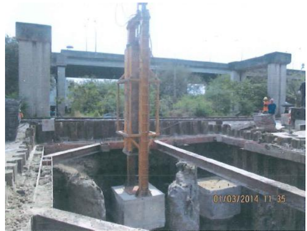
Fig. 6. Dynamic pile load test.
