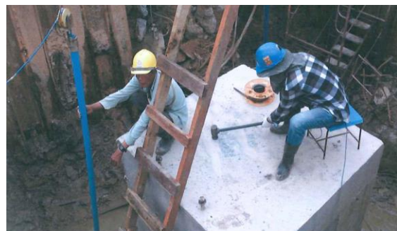
Fig. 4. Parallel seismic test on existing bored pile.
