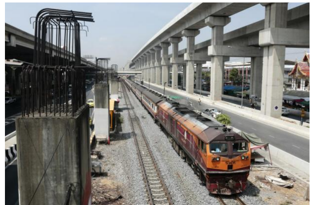
Fig. 11. Completion of SRT Red Line (elevated).
