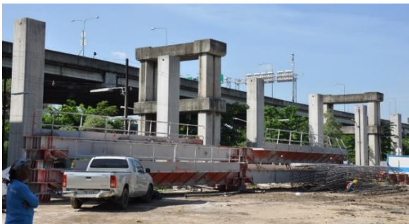
Fig. 2. Pillars along the current SRT Red Line.
