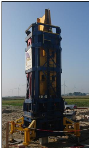
Fig. 6. StatRapid system positioned over the test pile.
