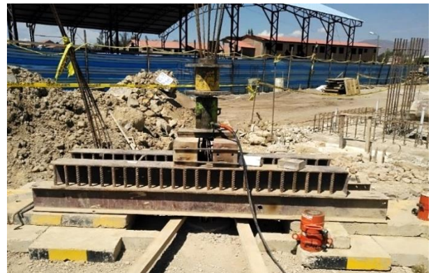
Fig. 5. Tension load test executed.
