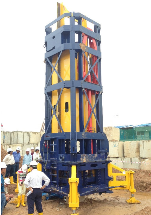
Figure 2. StatRapid System for Rapid Load Testing of Piles at Punggol C36 Project
