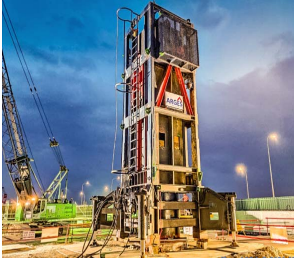
Fig. 2. Rapid load test impact hammer.
