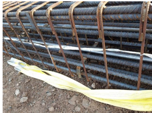
Figure 5. Wire placement in the cage.
