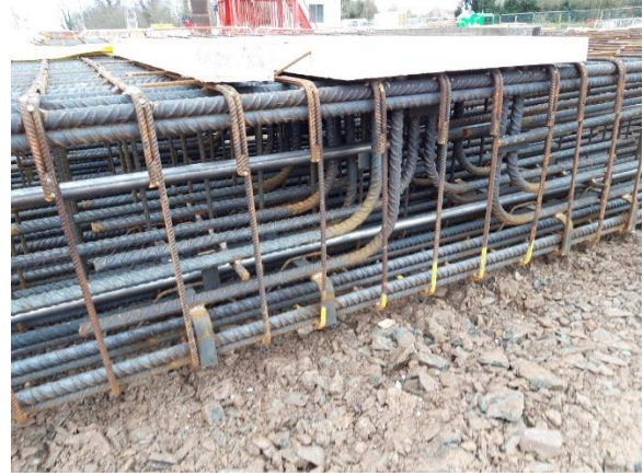
Figure 6. Cage with foamboard attached.
