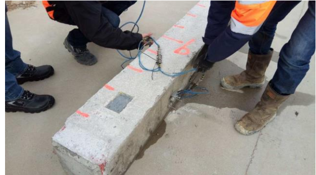
Fig. 3. Sensors placement for dynamic load test.
