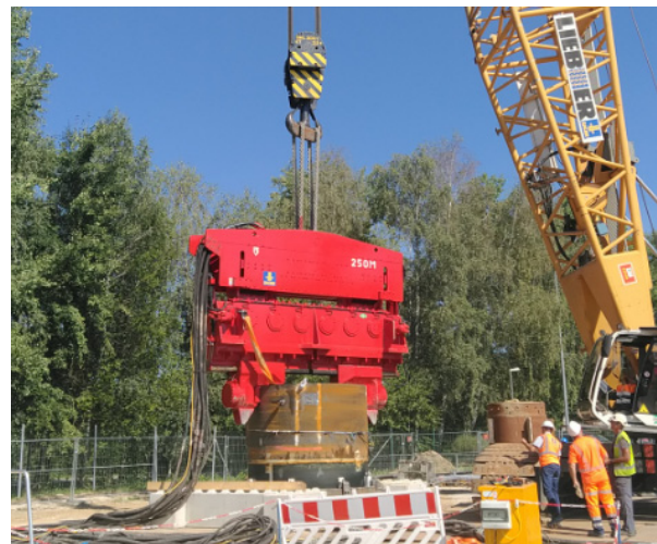
Fig. 3. OPT tests with 250 M PTC vibro – End of vibro drive.
