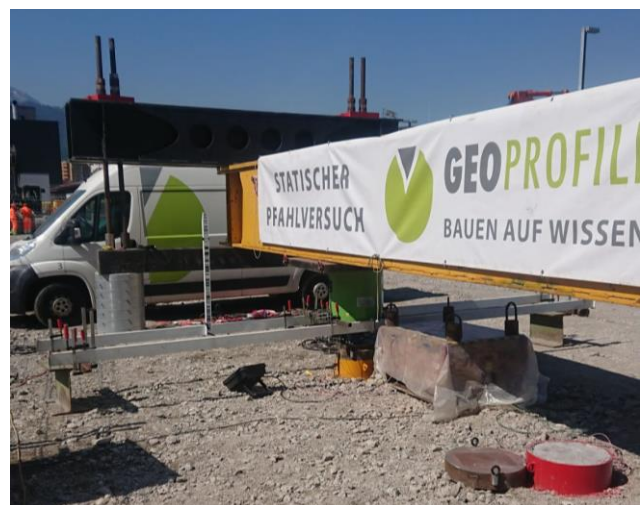
Fig. 5. Static pile load test with steel truss and reference beam
