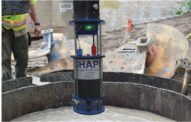
Fig 1. Shaft Area Profile Evaluator being lowered into a drilled shaft excavation.
